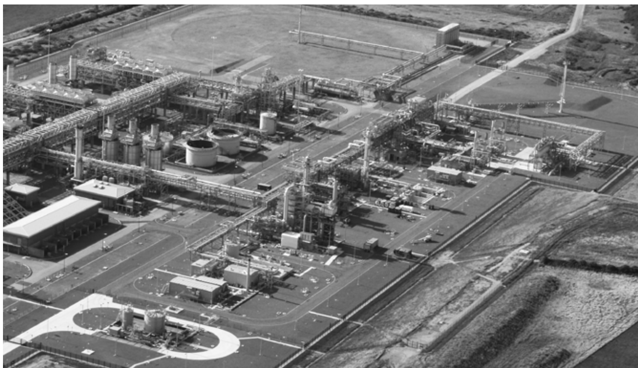
Harbour Energy's UK river terminal
